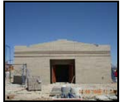
Storm Shelter during construction
