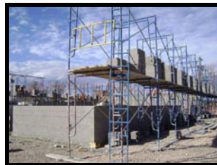
Project site during construction
