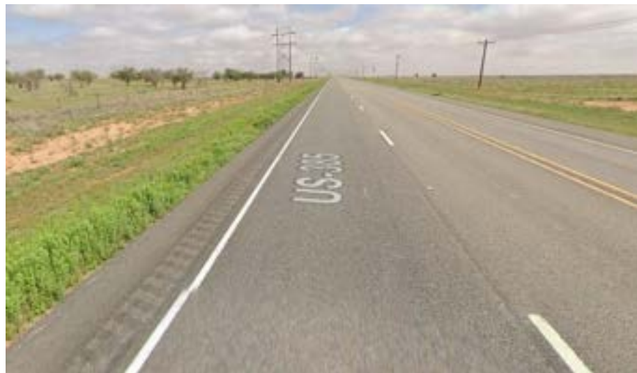
Figure 5. Super 2 Alternating Passing Lane (Source: Google Earth)
