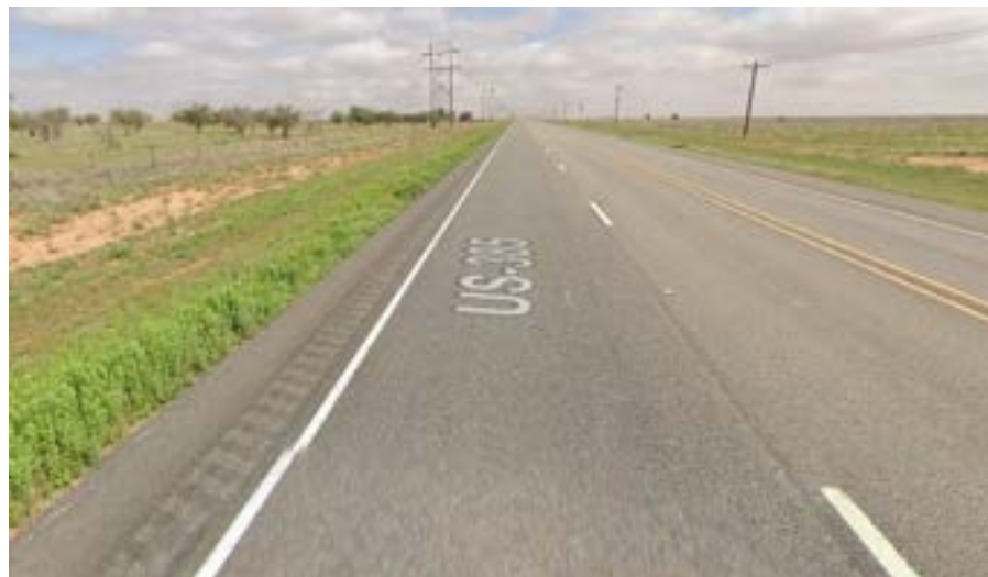
Figure 3-4. Super 2 Alternating Passing Lane (Source: Google Earth)
